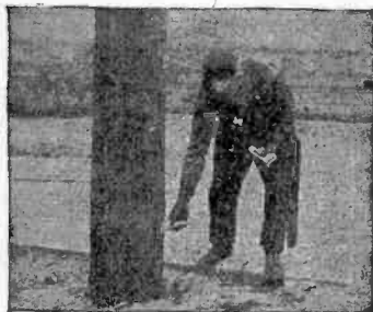
FIG. 5,844.—Installing Pierce detachable step. Step 3. The lineman attaches the steps as he climbs the pole.
