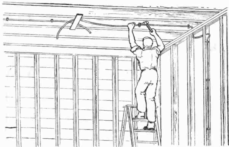
FIG. 5,450.—Non-metallic sheathed cable run parallel with beams.
