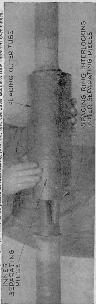
FIG. 6,070.—Assembling Conducell. Second operation: Placing the outer seamless tube over the inner separating pieces which have previously been placed in position and locked by the spacing rings.
