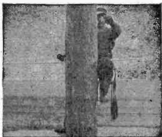
FIG. 5,844.—Installing Pierce detachable step. Step 3. The lineman attaches the steps as he climbs the pole.
