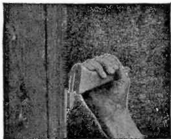
FIG. 5,842.—Installing Pierce detachable step. Step 1. Slip the plate over the lag and drive the lag screw until the plate bites into the pole.
