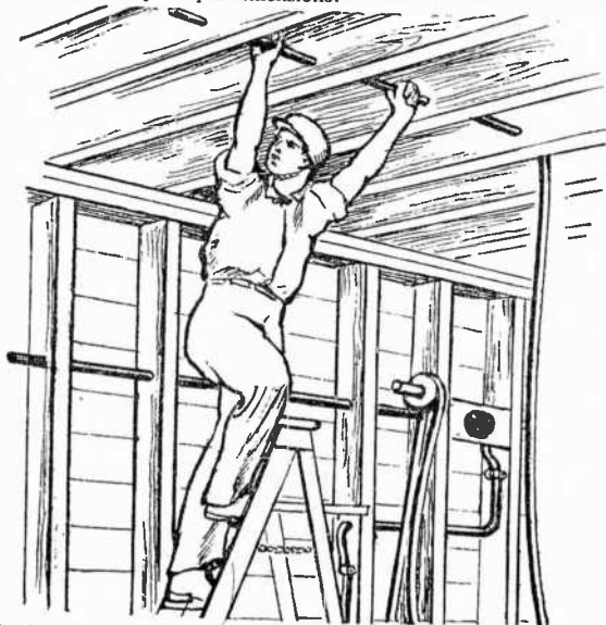
FIG. 5,444.—Passing non-metallic sheathed cable through holes bored in beams.
