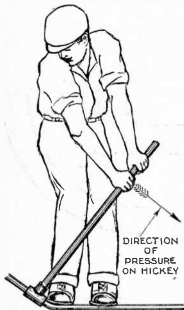
FIG. 5,515.—Method of bending conduit with a hickey. In bending , the conduit to be bent is placed on the floor and the tee slipped over it. The workman then places one foot on the conduit close to the tee, and pulls the handle of the bender toward him. As the bending progresses, the workman should take care to continually move the bender away from himself, to prevent duckling of the conduit.
