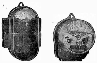
Fig. 4,513.-General Electric single phase watt hour demand meter.
