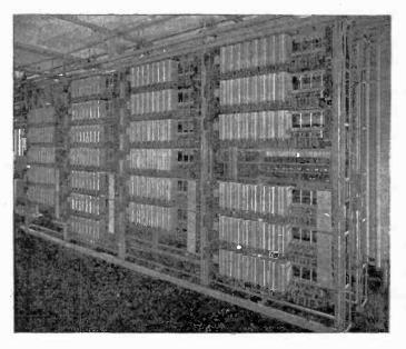
FIG. 7,663.-Step-by-step connectors mounted on switch frames.
