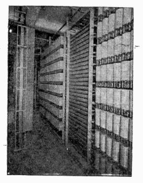
FIG. 7,674. -Groups of selectors mounted on switch frames.
