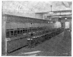
FIG. 7,571.-Large manual P. B. X switchboard.
