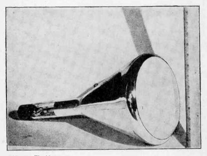
FIG. 10-The kinescope.
