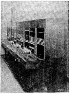
Fro. 7,570.—Multiple cord type P. B. X. switchboard of three positions. Note the dial on each position; this is made necessary since the P. B. X. is connected with trunk lines to a dial central office. The capacity of this switchboard without increasing the number of positions is approximately 500 lines.
