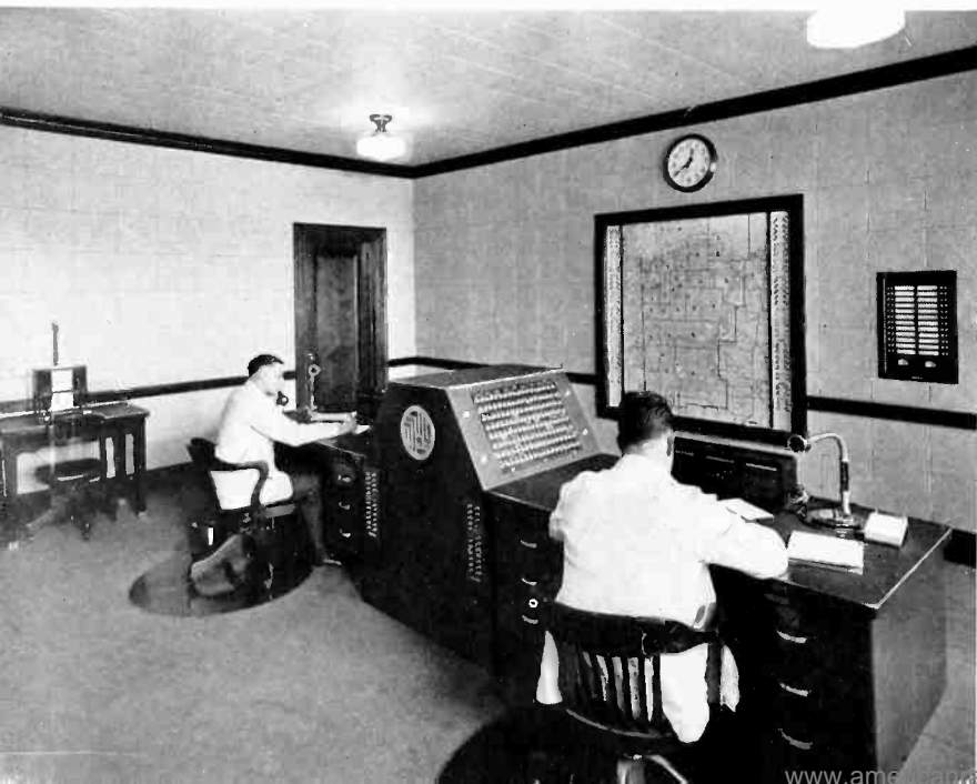
Dispatchers' studio. Keys in center of control desk operate car indicating lights on large wall map. Loudspeaker from output of remote receivers is located in the center of control desk.
