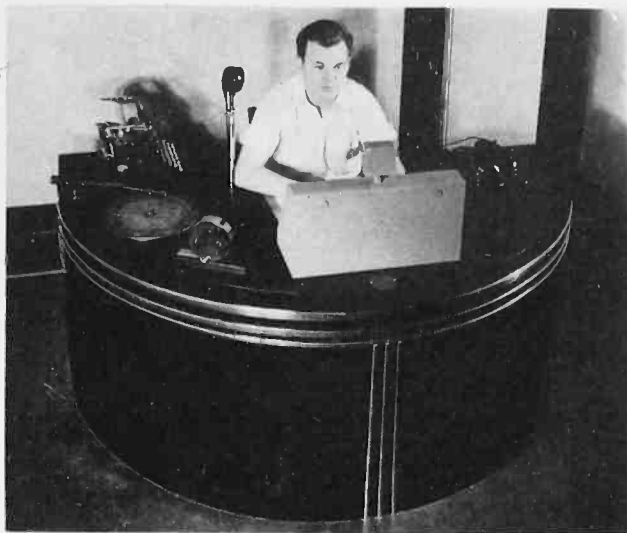
Control desk showing control assembly, rack, frequency monitor, turntable and temporarily installed microphone. Western Electric Non-directional microphones are used in WCLO's new studios.
