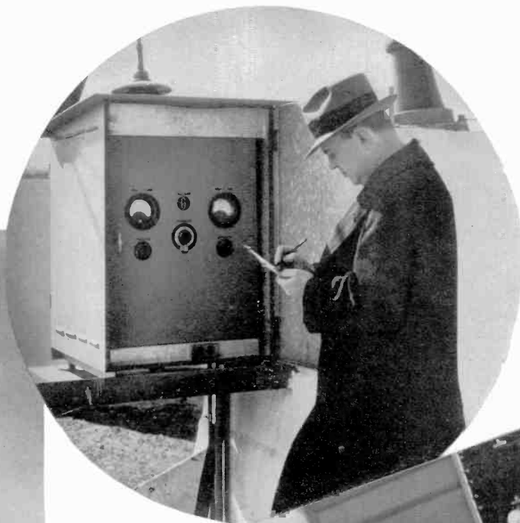
The antenna coupler unit— Windham checking antenna current
