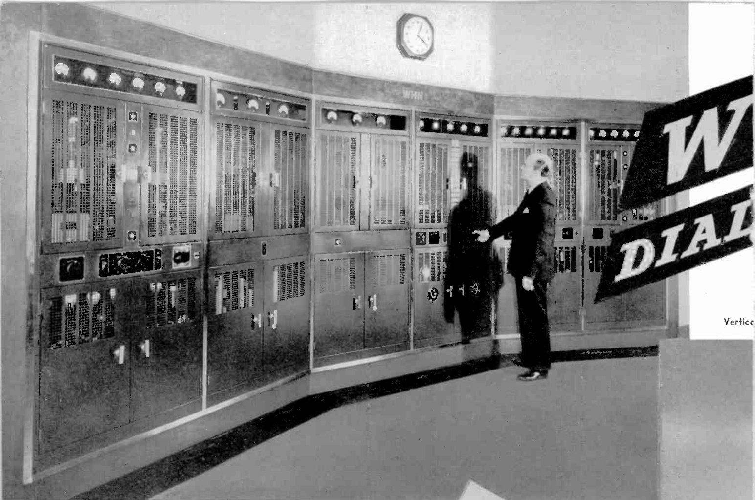
Gordon R. Windham, Chief Engineer, at the panels of 5 KW Transmitter. The two panels at the right comprise a Western Electric 1 KW Transmitter used for standby
