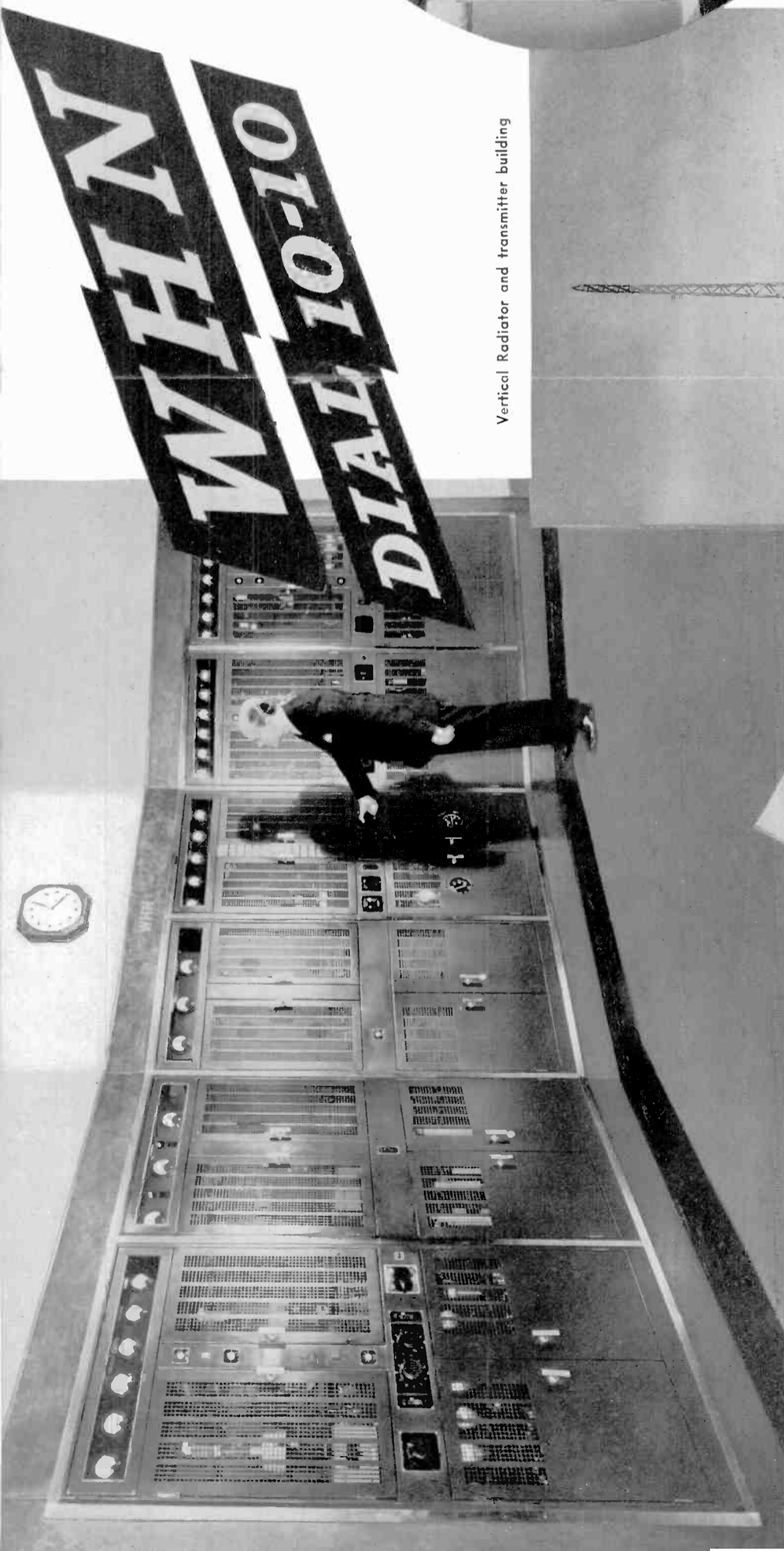
Gordon R. Windham, Chief Engineer, at the panels of 5 KW Transmitter. The two panels at the right comprise a Western Electric 1 KW Transmitter used for standby
