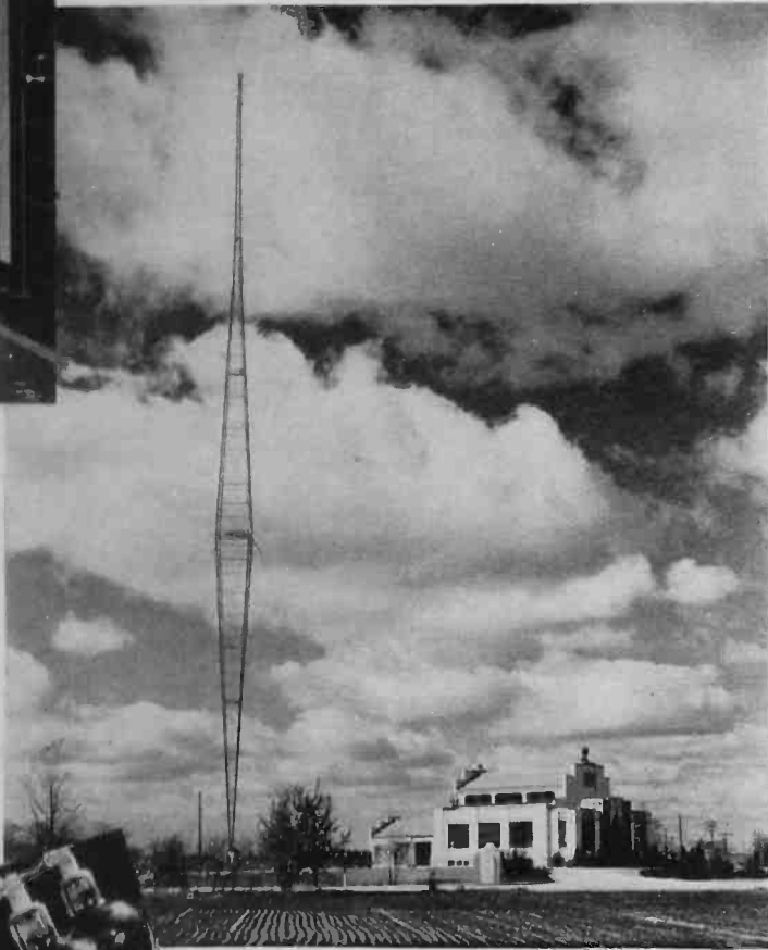
The 733-Foot Single Mast Radiator and Transmitter Building
