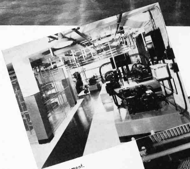
Panel layout of Western Electric 50,000 Watt High Fidelity Transmitter.
