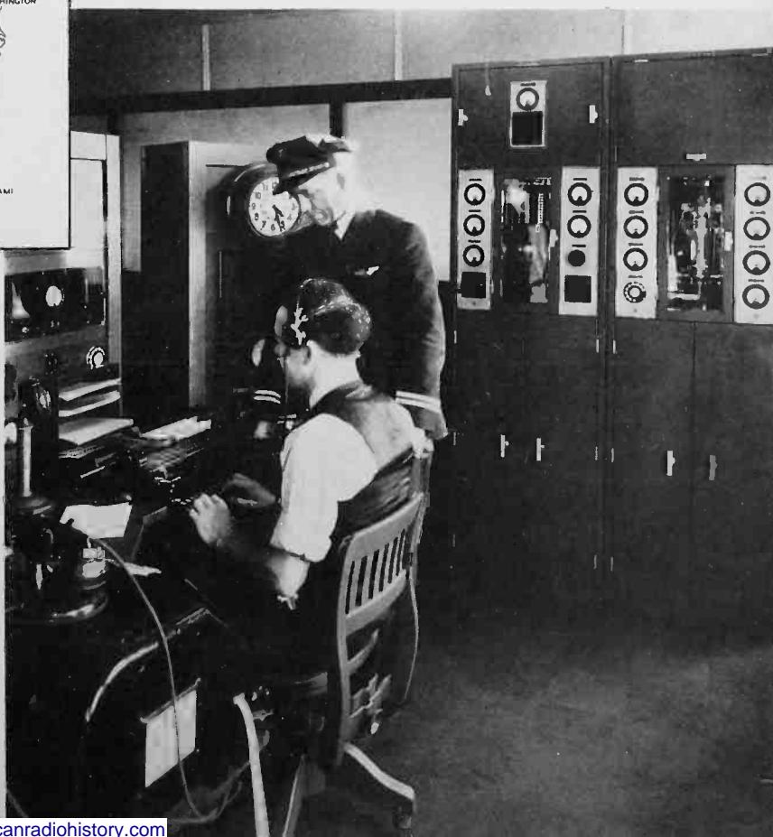
Radio ground station of Eastern Airlines at Newark Airport. E. L. Saunders, radio operator, is typing a message for Fred A. Jones, pilot. In the background is the Western Electric 400 Watt Transmitter. To the left is a cabinet containing control equipment and loudspeaker for the receiver, and next to this is speech amplifying equipment.
