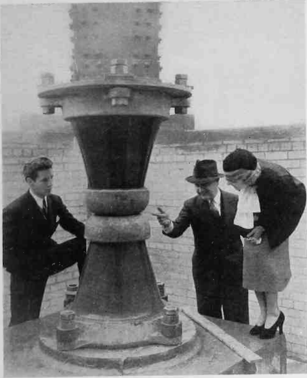
Leo Fitzpatrick shows the porcelain tipped base of WJR's 733-foot single mast antenna to two interested spectators.
