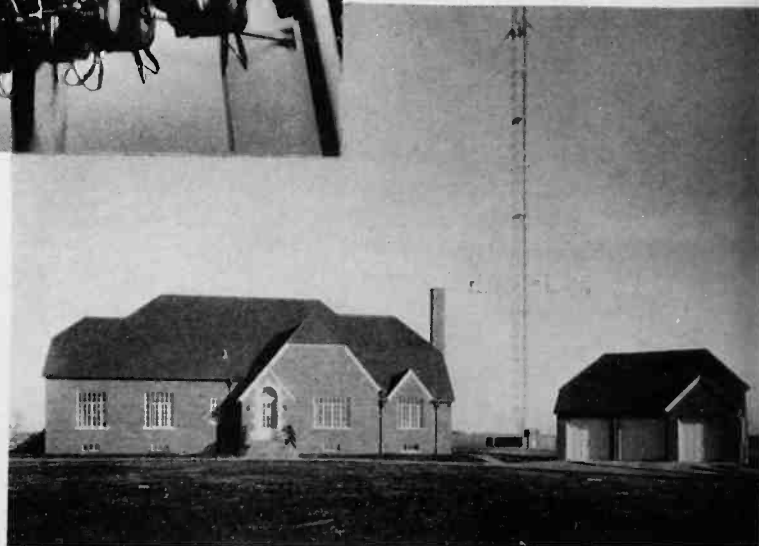
The transmitter station and five-room home for the resident operator.
