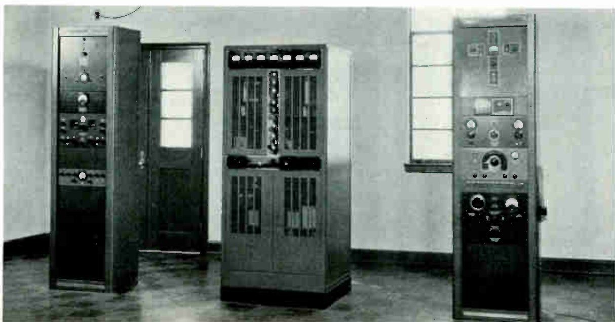
Control room showing Western Electric speech input console, turntables and audition controls. Left: Engineering staff — Carl Delay, Chief Engineer Gladman Upchurch, Donald Brooks.
