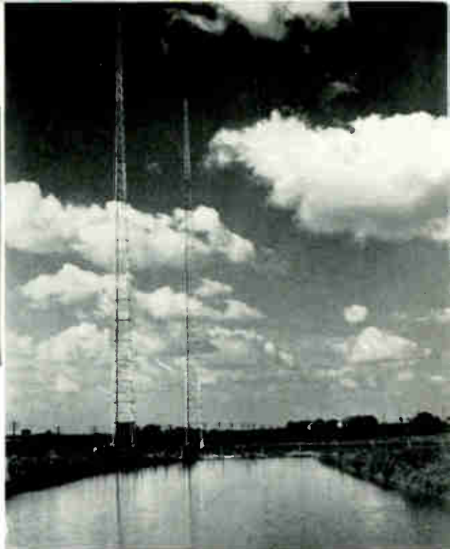
These towers comprise the directive antenna system.
