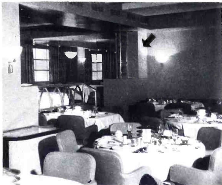
Here is a corner of the main dining room. Arrow points to one of six well-concealed loudspeakers which provide diners with music.
