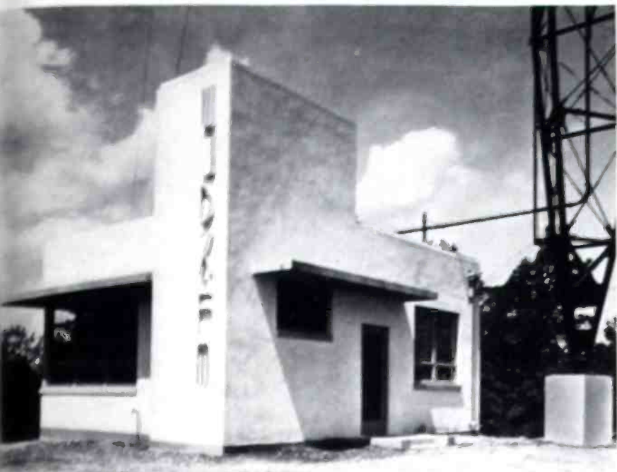
New transmitter building five miles from city houses 10 kw FM transmitter for WJDX-FM, with base of antenna tower visible at right.
