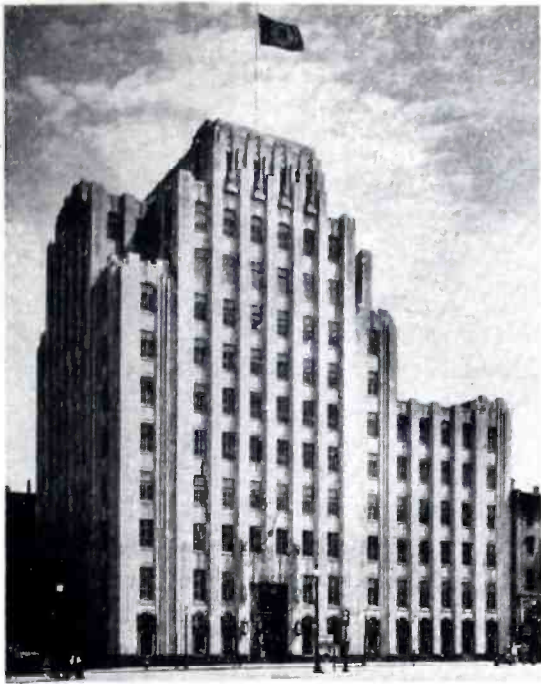
Boston terminal of radio relay system: the Bowdoin Square building of New England T. and T. Co.
