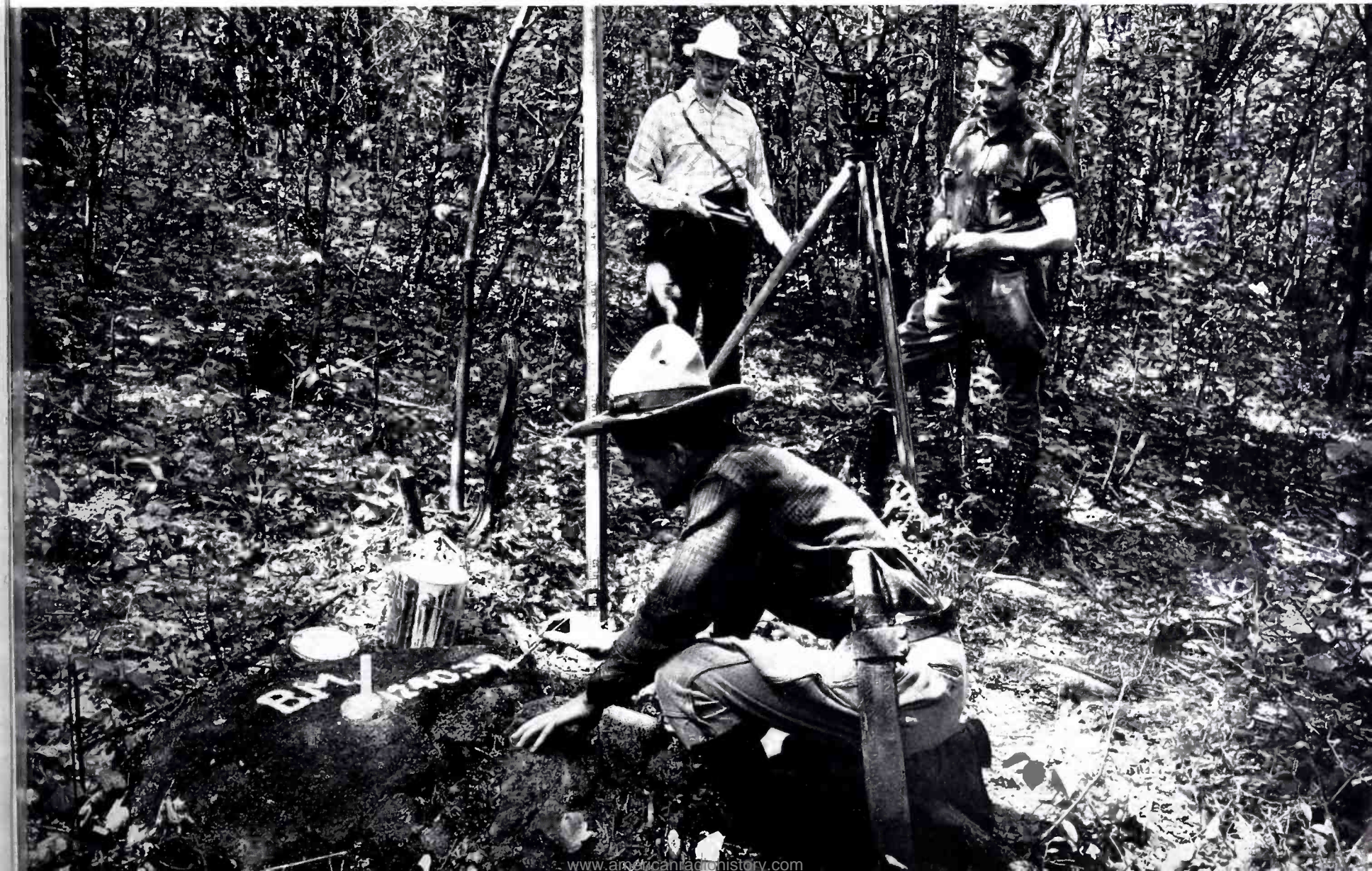
Surveyors establish a bench mark on a rock on Jackie Jones Mountain, site of first of seven radio relay stations along A. T. and T.'s radio relay system
