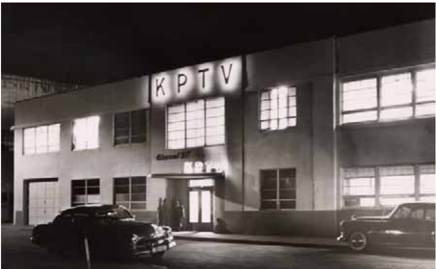
Night photo of KPTV studio building. Note the "Channel 27" above the entry way.
