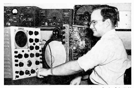
Fig. 5. Mr. Garner is shown using a laboratory oscilloscope to check wave-forms in a Stromberg-Carlson Model TV-12 Television Receiver.
