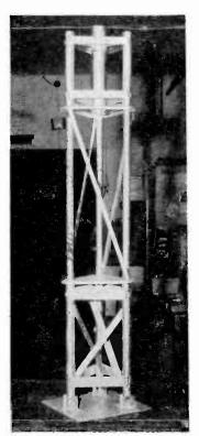
Fig. 2. One section of a typical television antenna tower. Used for heights above forty feet.
