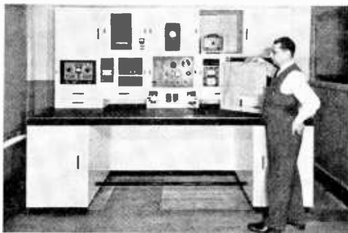
George J. Rohrich, Engineer in charge of the N. R. I. laboratory, points to one of the spring catches which hold the instrument panels rigidly in position, yet make them instantly removable.
