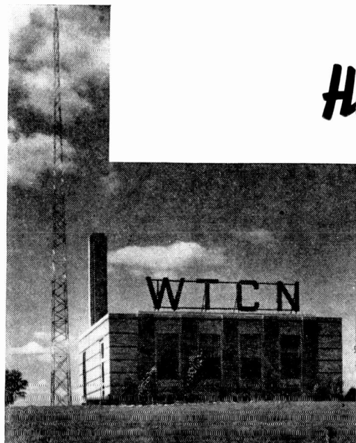
Single mast antenna and transmitter building, located equidistant between the Twin Cities.
