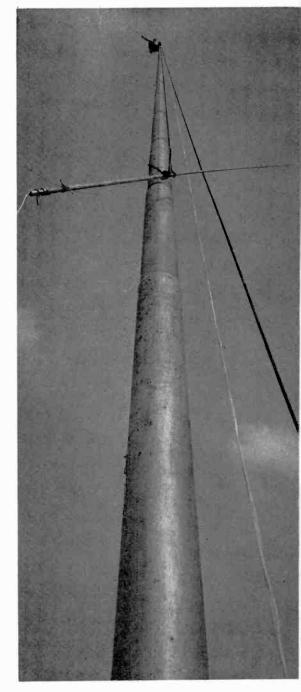
Steeplejack erecting antenna of Newark Police Radio. 22 foot brass tube is being installed on top of 100 foot flagpole. Antenna tube is 600 feet above ground.
