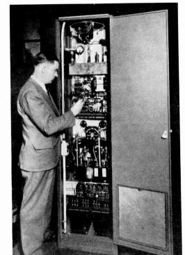
Inserting a tube in rear of the transmitter of Police
