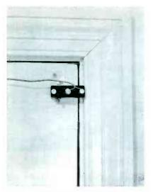
Fig. 7. Microswitch installed on door.
