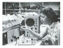
FIG. 9. Helen Gillespie of Assembly pre-adjusts the trimmers to be used in a CONAR 280 Signal Generator kit. Proper adjustment produces a circular pattern on the scope screen
