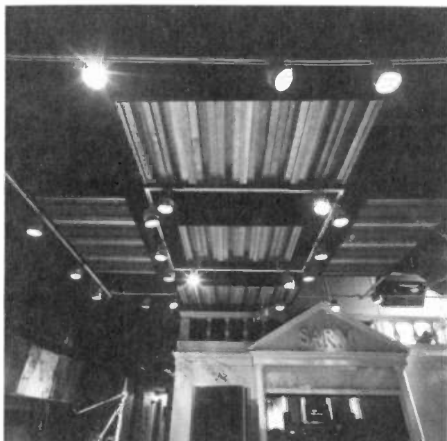
Figure 11. Suspended ceiling mounted RPG diffusers at (Top) Blue Jay Recording Studios, Carlisle, MA. Acoustical consultant Russell E. Berger. (Bottom) SARM Recording Studios, London, UK. Acoustical consultant Neil Grant, DRL London. Ceiling systems integrate diffusion, absorption, and lighting.
