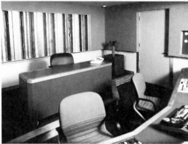
Figure 9. View of the RPG diffused rear wall in RFZ/RPG control rooms at (Top) Red Bus, London, UK. Acoustical consultant Neil Grant, DRL London. (Middle) Weik Music Group, Nashville, TN. Acoustical consultant Bob Todrank, Valley Audio. and (Bottom) San Francisco Production Group, San Francisco, CA. Acoustical consultant Randy Sparks, RLS Acoustics.
