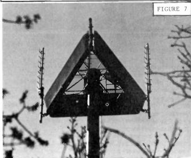
Many AM engineers have been surprised by the sudden appearance of a Cellular radio tower nearby.
