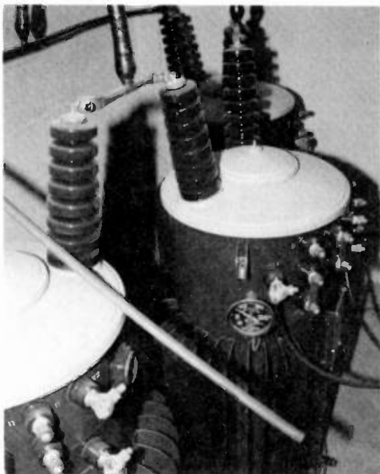
Liquid-filled Transformers
