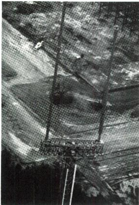
Fig. 8. Tee bar antenna support platform for two TV antennas.
