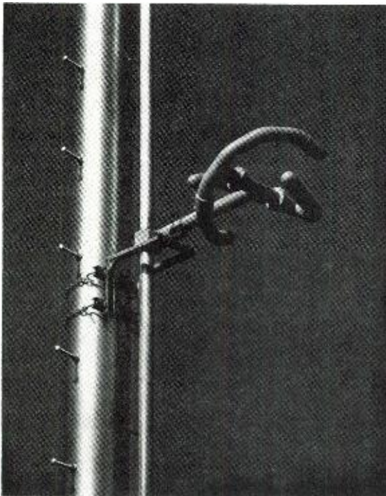
Fig. 10-A. Series fed element of Harris model FMXH non-symmetrical antenna. Typical pole mounting with rigid inter-bay coaxial feed line. (Photo courtesy Harris Corp.)
