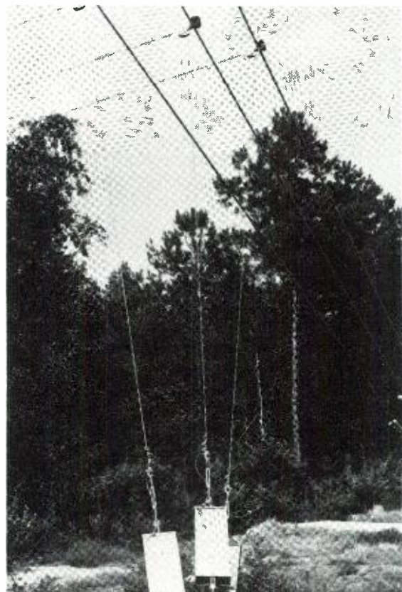
Fig. 6. Anchor connection with snubber system to prevent galloping.
