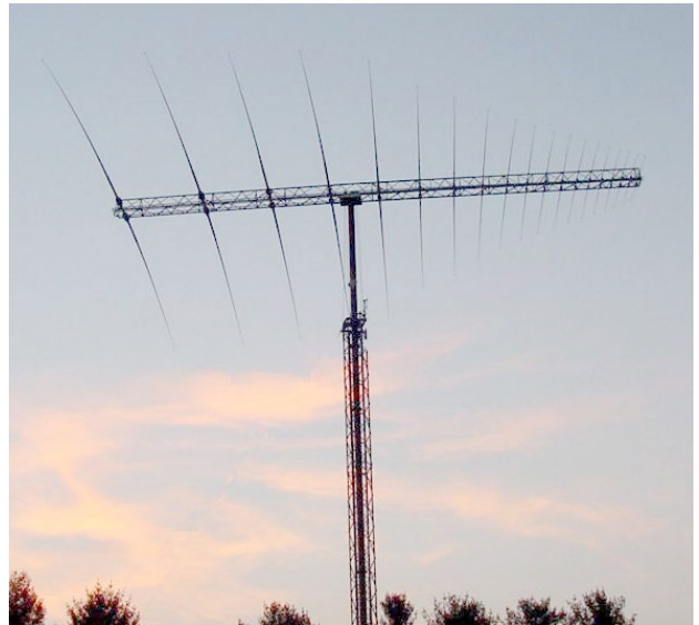
U.S. Antenna log-periodic dipole array delivers 7.0 dB from 13 to 30 MHz. (Courtesy: U.S. Antenna)
