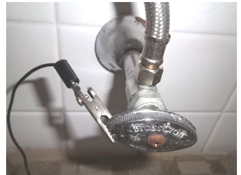
Water pipe - not as convenient but a good ground anyway, assuming you've got copper water pipes. This doesn't work with PVC.
