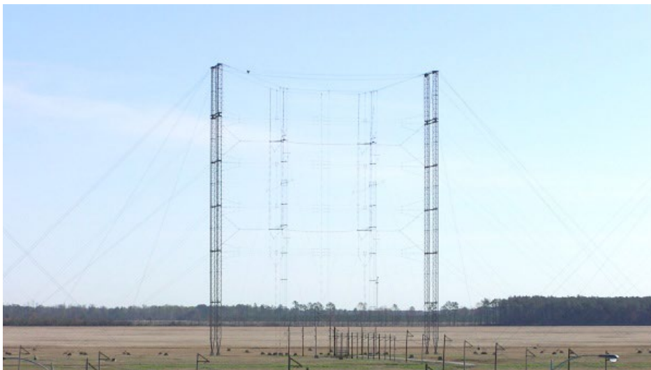
VoA Greenville curtain array delivers high power HF to a fixed point. (Courtesy: BBG Strategies)
