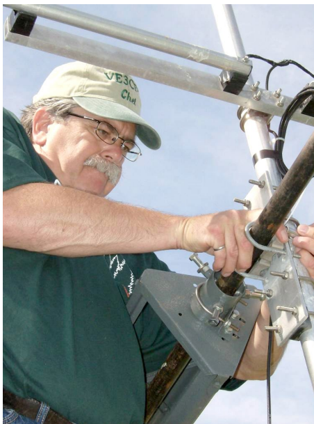
Chet Lataweic VE3CFK assembles an HF beam antenna for the 2009 Lambton County (Canada) Radio Club's Field Day.
