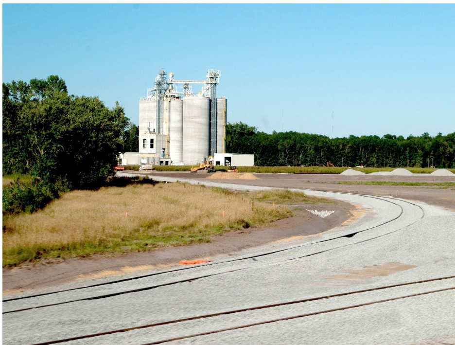
This new feed mill near Kinston, in eastern North Carolina required an unloading loop of about a mile of track, which had just been completed in 2010 when this photo was made from a passing train. The mill has since been receiving trains of up to 60 cars of grain.
