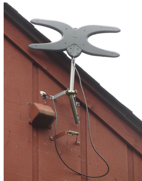
Gable mounted SKY-HDTV antenna. Of the old antenna supports needed for the previous antenna, only one is needed for the extremely lightweight SKY-HDTV antenna. A longer replacement mounting pipe will put it higher above the roofline. (Courtesy: Author)
