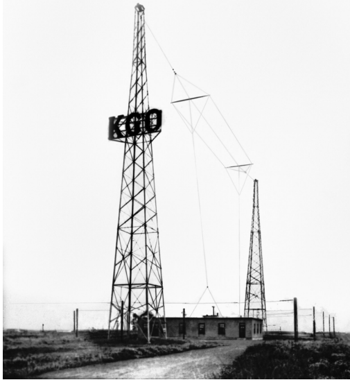
This photo shows the KGO transmitter building and antenna which operated from 1924 to 1947 at 5441 E. 14th Street in Oakland, on the grounds of a General Electric transformer factory. The two 150-foot steel towers that supported the antenna straddled the transmitter building, one on each side, at a spacing of 260 feet, so that the antenna was strung directly over the structure. Twelve counterpoise wires were strung parallel to the antenna fourteen feet above the ground and covering an area of 150 x 300 feet.
