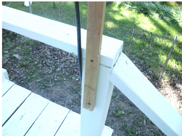
The 1x2 deck-screwed to a corner post of my back porch balcony.
