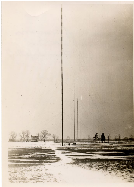
View of the main aerial system with horse and wagon near the base of one mast, human figure in Jacob's seat about half way up the mast. Flanges on the mast foundations were almost 6 feet wide. Photo taken in 1914 by Mr. Edward Henderson used by permission of the family of Edward Henderson.
