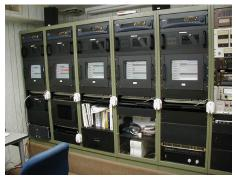
Controls for new 250,000 watt, DRM-capable, Thomson transmitters at TRW's Guam site. (Courtesy: TRW)
