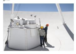
Above is the entry point to the horn antennas/detectors. Notice that the cluster of horns are offset, aimed upwards toward the secondary reflector above. Each horn is designed for operating on different bands. The little lamps are heat elements to dispel ice and frost and even rain drops. It has been known to happen even out in the desert. We climbed up a ladder onto the surface of the dish through a trap door near the ladder.
