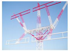
Thomson rigid dipole antenna, a "smaller" version of the large antenna on the cover.
