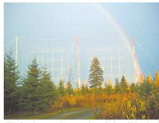
The Sterba curtain array is a chain of identical collinear elements as in the TCI Dipole Array at KNLS, Anchor Point, Alaska. The initial elements are shown here as a center-fed antenna, although it can be fed at other points as well. (Courtesy: World Christian Broadcasting)
