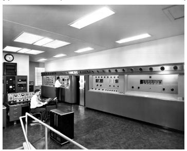
A view of the KGEI transmitter operator's position sometime before 1950. The original 50 kW transmitter is out of view at the left. To the right is the big 100 kW General Electric shortwave transmitter that was provided by the government during the war and broadcast as KGEX. (Photo courtesy of FEBC International)
