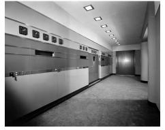
KWID's new 100 kW General Electric transmitter is shown installed and ready to turn on; February, 1942. (Photo courtesy of FEBC International)
