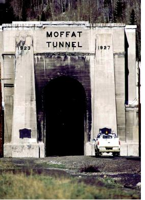
A signal maintainer in a hi-rail truck prepares to enter the almost seven-mile-long Moffat Tunnel in central Colorado. The single-track tunnel runs under the Continental Divide and contains a variety of safety equipment, including a continuous repeater antenna (for voice and radio control of remote locomotives) and equipment defect detectors
