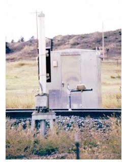
Wayside scanning equipment for reading RF tags on railcars and locomotives. The small box on the inverted L-shaped arm is the transmitter. The larger antenna on the vertical post reads the signals that are returned. The angle of the photo makes it look like the transmitter unit is between the rails. It is not.
