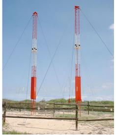
WWVH 15 MHz antenna array: Two half-wave vertical dipoles separated by a quarter-wave length and driven 90 degrees out of phase. (Courtesy: NIST)
