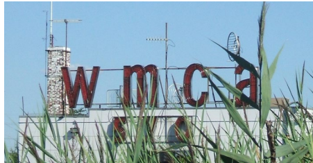
WMCA-570's transmitter building in New Jersey.
