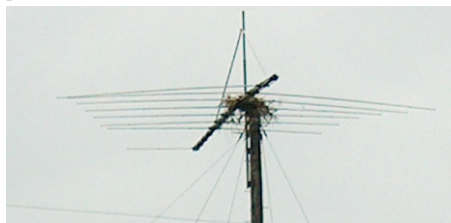
Figure 11 - WCC tower with log periodic antenna and bird's nest! (Look carefully at the center of the boom.)
