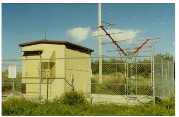
"V" shaped antennas at many longwave sites are for a separate 75 MHz marker beacon. This one is at LH/334 kHz, Bloomington, IL.
