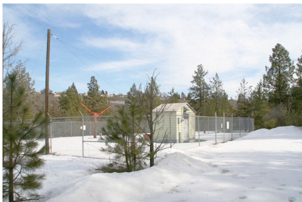
Beacon GE/388 kHz, Spokane, WA. Note the V-shaped antenna to the left of the building. This is for a separate 75 MHz marker beacon. (Photo courtesy of Kriss Larson)
