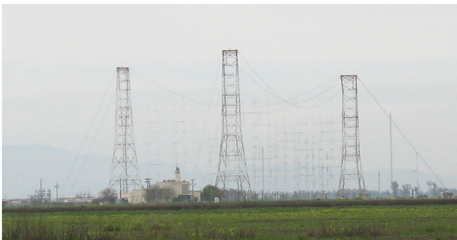
Figure 1 - The former Voice of America Relay Station in Dixon California from a distance.
