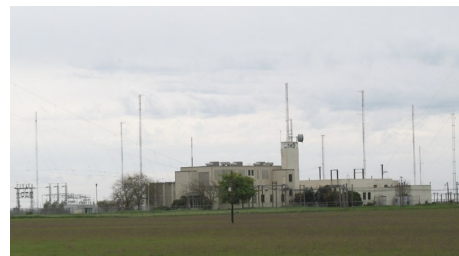
Figure 3 - Although the facility closed sometime ago, you can still see the rhombic antennas in the background.
