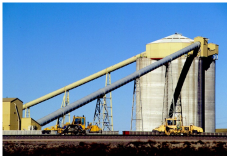
Track maintenance machines (ballast regulators) in front of the loading silos of one of the Powder River Basin mines. Behind them, on a lower level, a coal train is on the loading loop of the mine.
