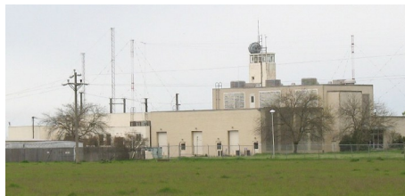
Figure 7 - VOA Dixon Relay Station from another angle.
