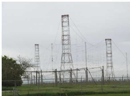
Figure 5 - Dipole arrays consisting of rows and columns of dipoles known as a curtain antenna. These antennas are rated up to 500 kilowatts.
