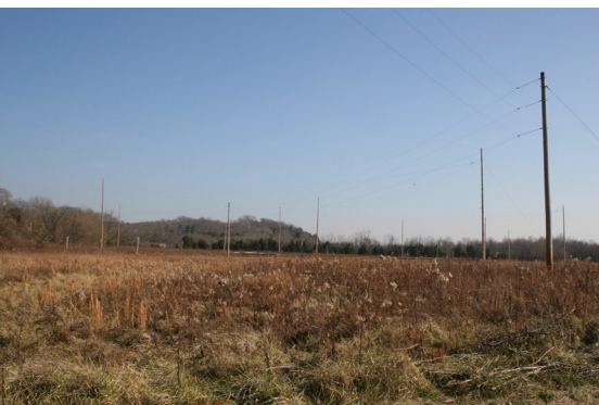
Not a power line installation but a big time Rhombic array antenna at WWCR’s antenna farm. This, along with its 100 kW transmitter, accounts for its needle bending signal strength across North America. Look for plenty of real estate if you plan this type of antenna for your own HF broadcast station. (Photo by Cameron Keel courtesy WWCR)
