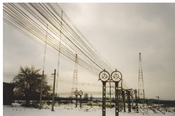
Stretching out to the western portion of the antenna farm, these transmission lines handle both MW and SW chores.
