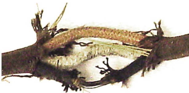
One of many worn spots in the line cord reveals frayed wiring. The asbestos-covered lead in the center is the resistance element.
