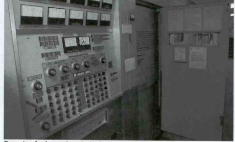
Transmitter four's control panel, with the door open for frequency changes
