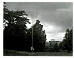
The self contained 10 watt AM radio station KFQ-70 has a typical range of 4-6 miles. Tower height is 49 feet. Photo, courtesy NIH.
