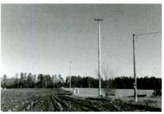
Mike Leahan (WI) sent this photo of SLY (344 kHz) near Hayward, WI. Although not visible here, the antenna consists of two parallel wires strung between the cross-arm utility poles. The shed houses the beacon transmitter.
