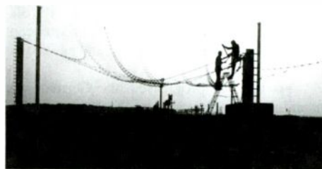
Antenna work at Wertachtal transmitting station, Courtesy: DW Foto Archiv
