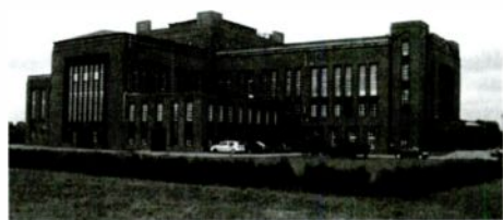
The main transmitter building at Nauen, now restored. Courtesy Wumpus
