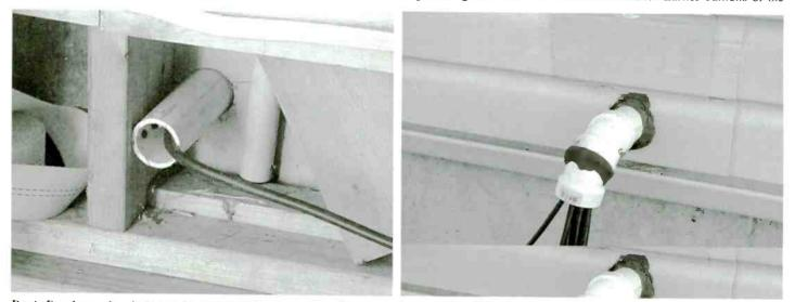
Denis Dandeneau's solution to the antenna lead-in problem. Easy to find and work with, PVC pipe is fitted through a hole cut with a low cost 2" hole saw that fits on your drill. (Courtesy Denis Dandeneau)
