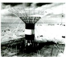
Example of a Cross Field Antenna similar to one which Music Mann 279 plans to use. The 9 meters high model is currently radiating 100 kilowatts from a site at Barnis is Southern Egypt, on 603 kilohertz (approx 495 meters Mediumwave)
