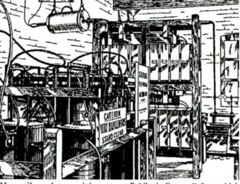
Marconi's spark-transmitting room at Poldhu in Cornwall, from which wireless signals were first sent across the Atlantic. The spark gap is in front of the window on the right.
