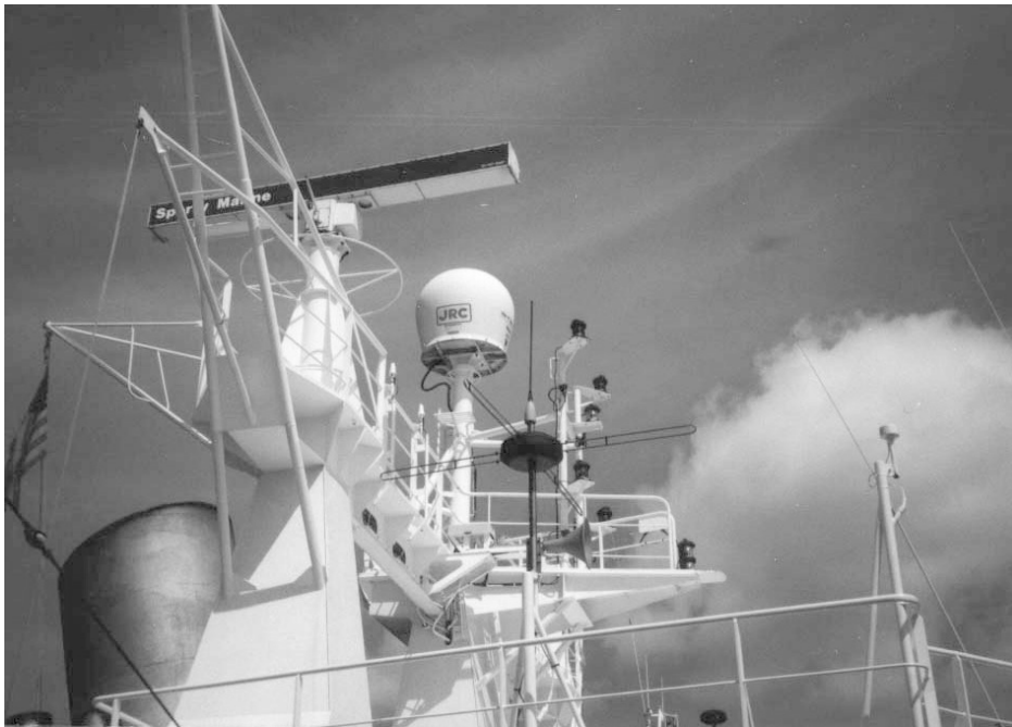
Radar mast, APL Singapore
