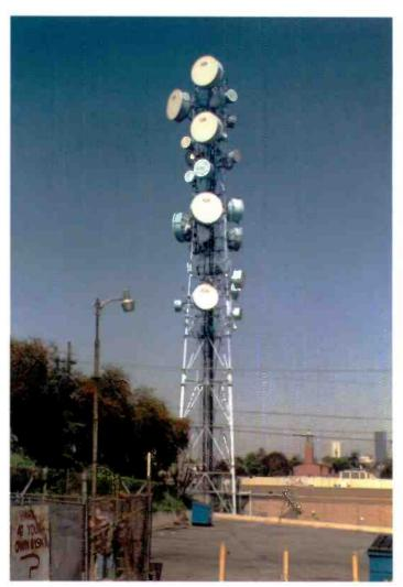
While it would be tempting to say this is an all-weather test rig for kettledrums, in fact it's a microwave hub for a telephone network. The purpose is to combine thousands of telephone calls by multiplexing them on a microwave radio link rather than to have to provide hardwire lines for them. (Photo submitted by Al Shack, Simi Valley, CA)
