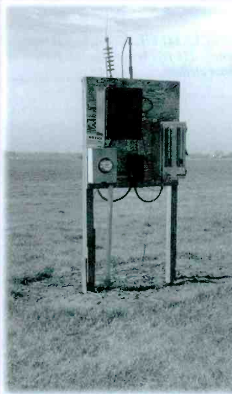
Winchester, IN, "AWW" 212 kHz. Transmitter is in small silver box, antenna matching unit is black box.
