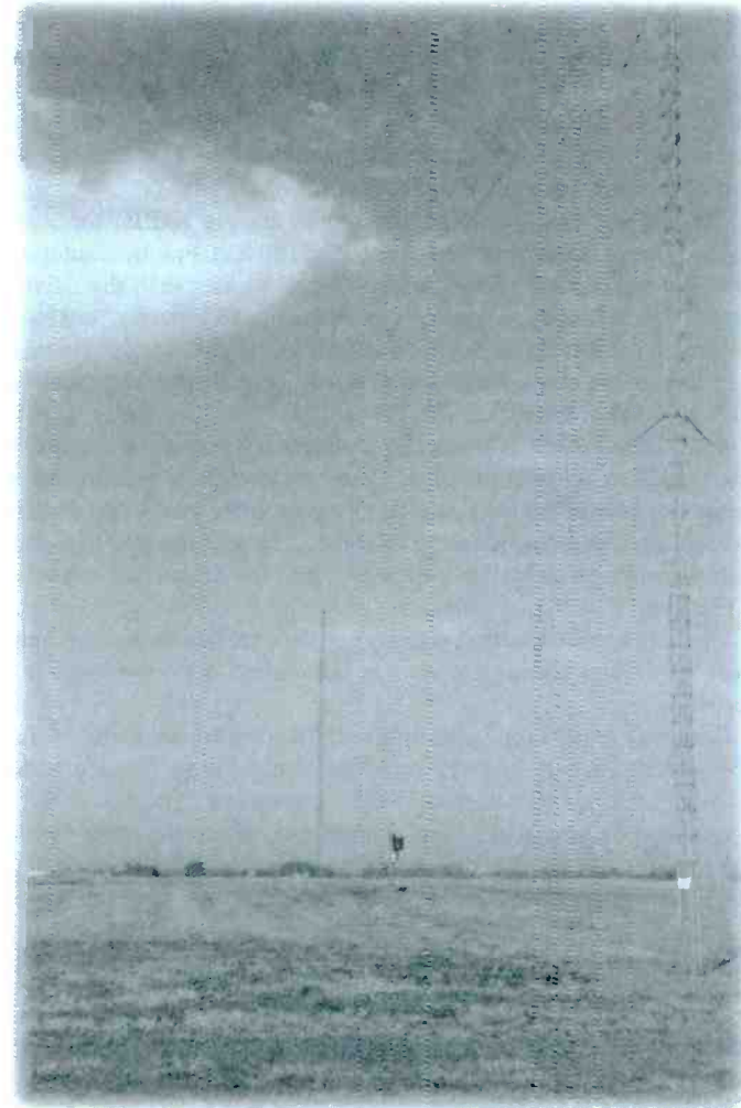
Winchester, IN, "AWW," 212 kHz. Privately owned, low cost, simplest type of MH. Equipment on exposed mount, antenna flat top "T" between TV type masts.
