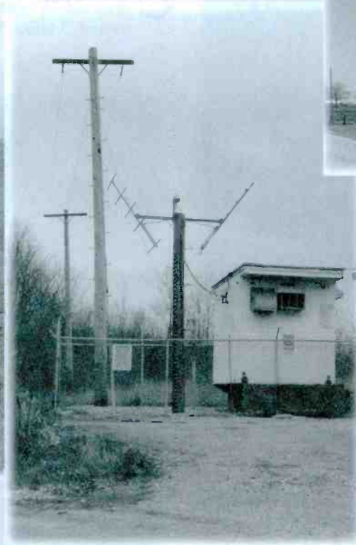
Dayton, OH, "AT," 315 kHz, LOM/OM. Old style FAA owned. Equipment in trailer. 50 foot flat top "T" antenna. "V" shaped Yagi array is 75 MHz OM antenna. "Bird house" on pole is monitor for OM.
