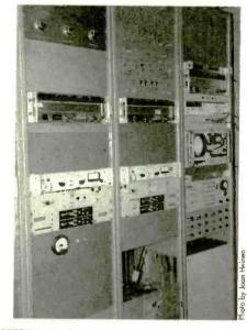
WWVB's clock RF oscillator, frequency counter and controller
