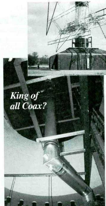
Each of the four new transmitting units at Nauen contains a 500 kW transmitter in a heavily shielded building and a rotatable antenna on its roof. The short path between transmitter and antenna keeps loss on the feeder line low and efficiency high. Everything can be remote controlled from a console in the main control room.
