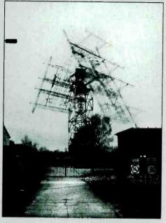
Germany's antenna technology of the past was impressive in its own right. Still the only one of its kind, the antenna built in 1964 for Radio Berlin International consists of two antenna arrays with rigid dipole units that can be used alternately depending on the frequency employed and the area to be covered. It can be rotated up to 360 degrees horizontally and tilted up to 50 degrees vertically.
